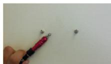
**3. Put screws "most of the way In" to anchors**
