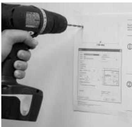
3. If using drywall anchors, set them into the wall. Then, drive the screws into the wall leaving a gap of about 1/8" (3 mm) between the screw head and the wall. If not using anchors, just drive the screws.
